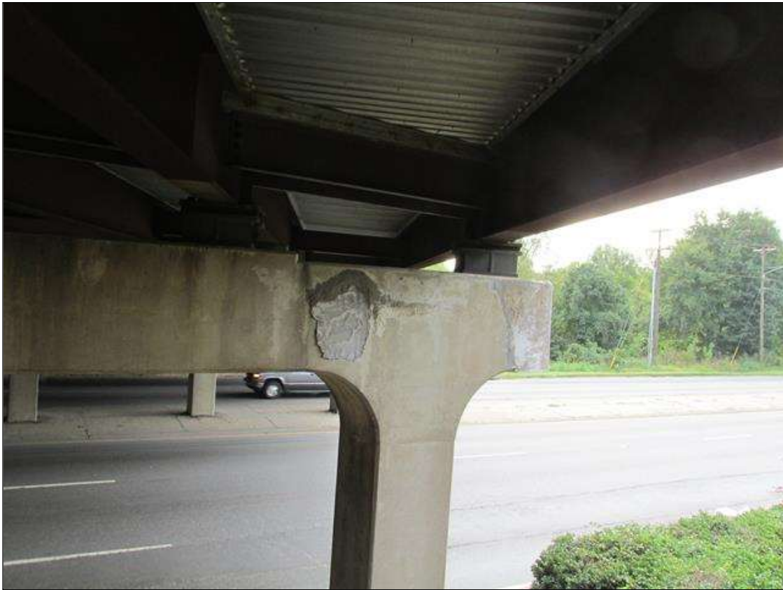
Bent 1 Cap : SPALL REPAIR
