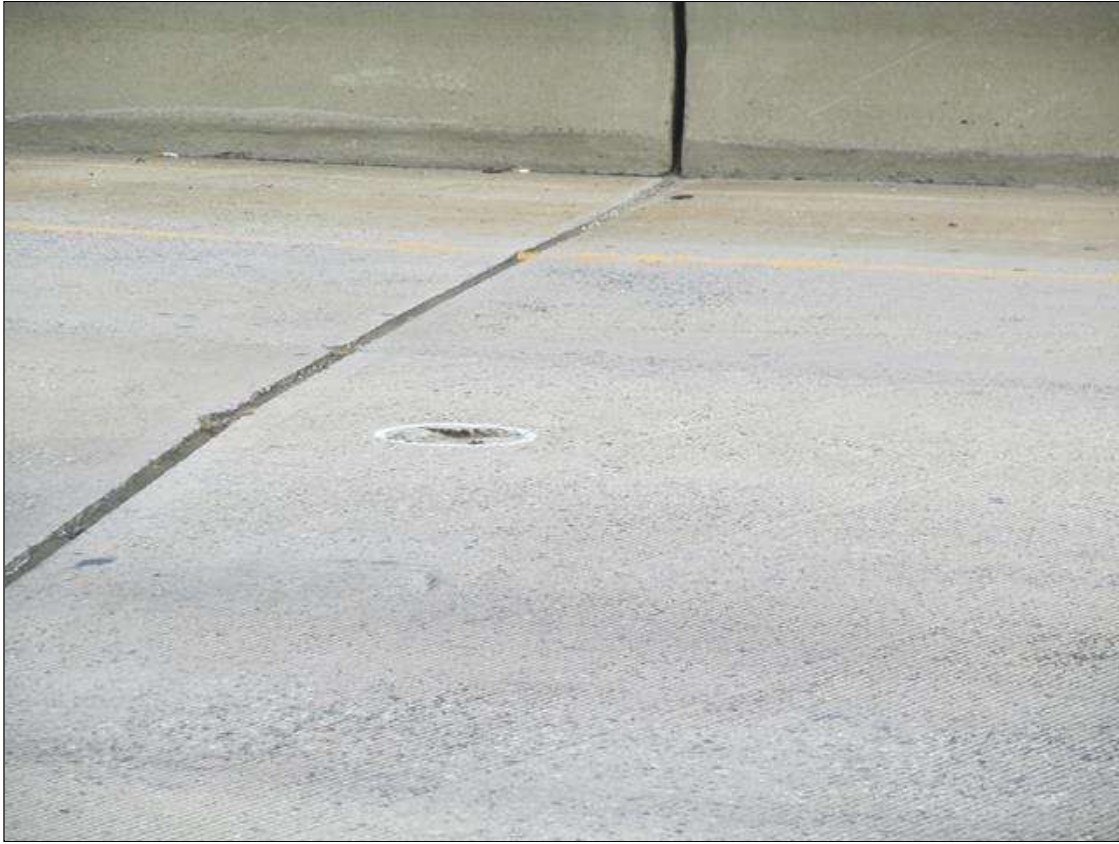
1 Square Feet of Delamination/Spall/Patched: Spall greater than 1 in. deep or greater than 6 in. diameter. Patched area that is unsound or showing distress. Does not warrant structural review.
