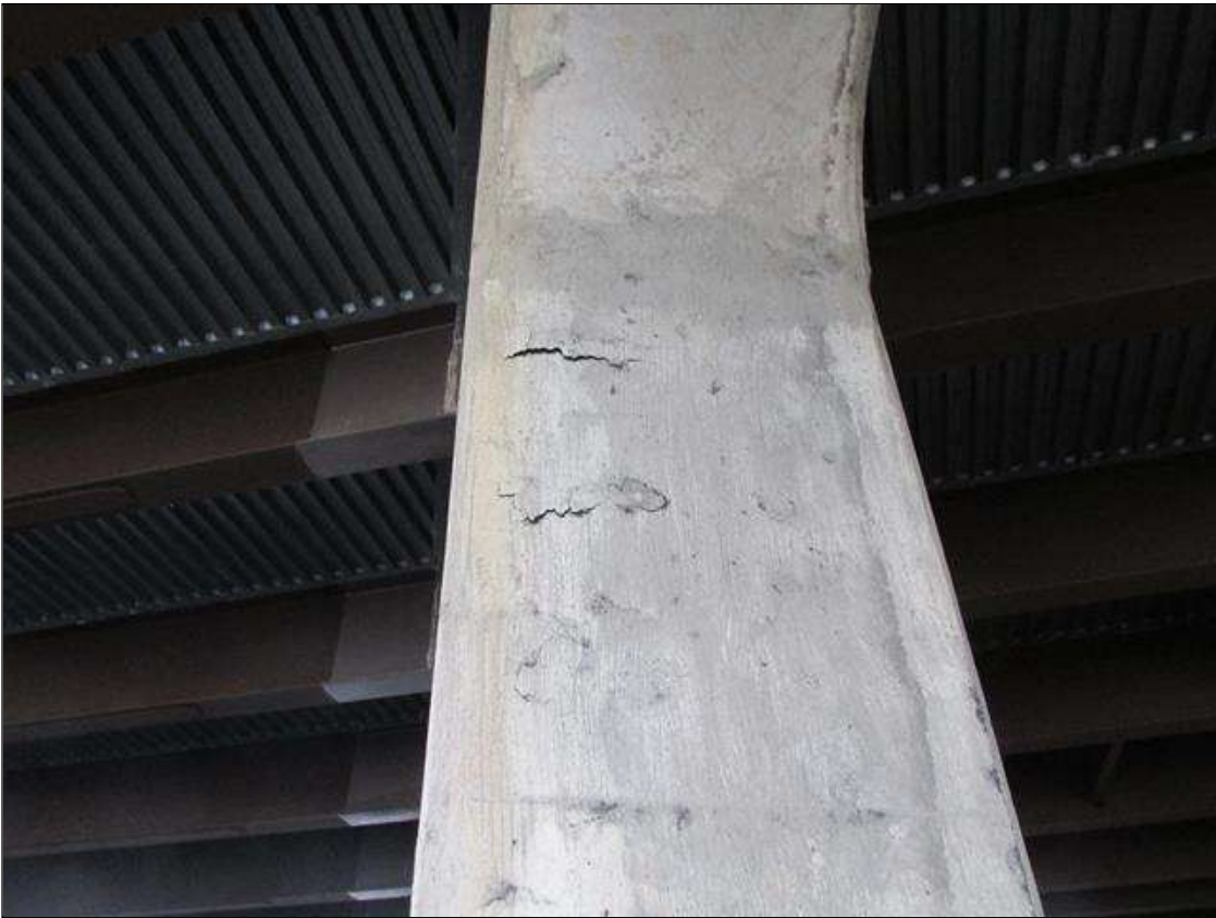
Bent 2 Pile 5: 1 Each of Delamination/Spall/Patched Area: Spall greater than 1 in. deep or greater than 6 in. diameter. Patched area that is unsound or showing distress. Does not warrant structural review.
