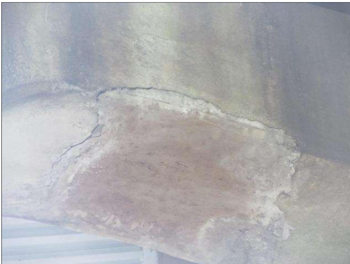
Bent 5 Cap : 6 Feet of Cracking (RC and Other): Width greater than 0.05 in. or spacing of less than 1 ft. SPALL REPAIR LOOSE.
