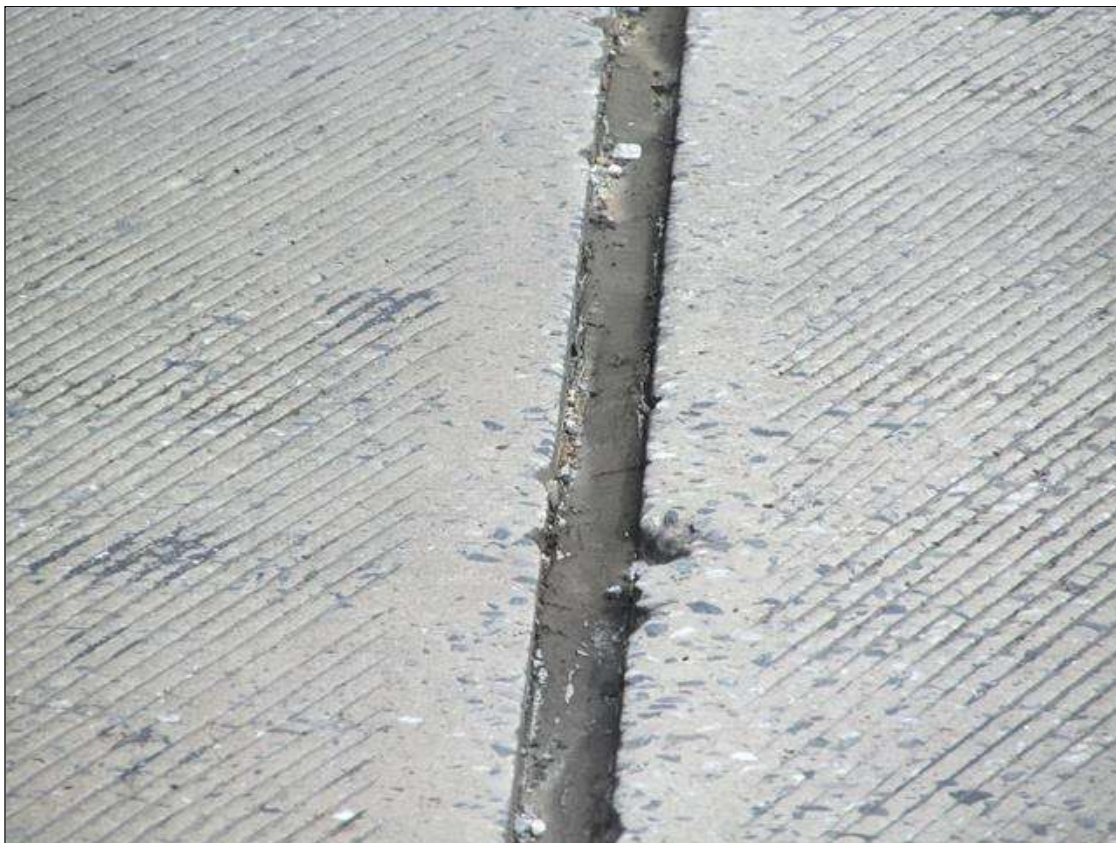
Expansion Joint 1 : 68 Feet of Seal Adhesion: Adhered for more than 50% of the joint height.
