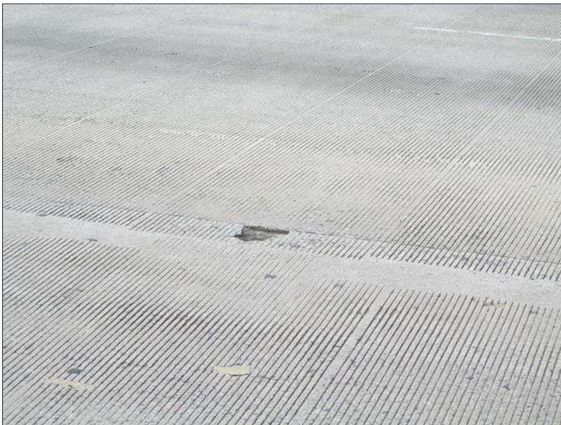
Span 2 Wearing Surface: 1 Square Feet of Delamination/Spall/Patched Area/Pothole (Wearing Surfaces): Spall 1 in. deep or greater or 6 in. diameter or greater. Patched area that is unsound or showing distress. Full depth pothole. NB LANES
