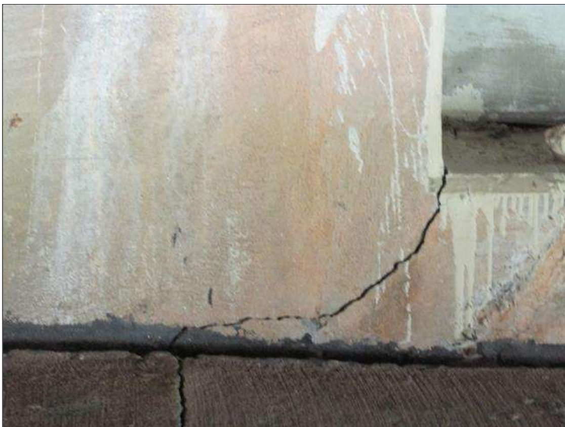
End Bent 2 Cap : 8 Feet of Cracking (RC and Other): Width greater than 0.05 in. or spacing of less than 1 ft.
