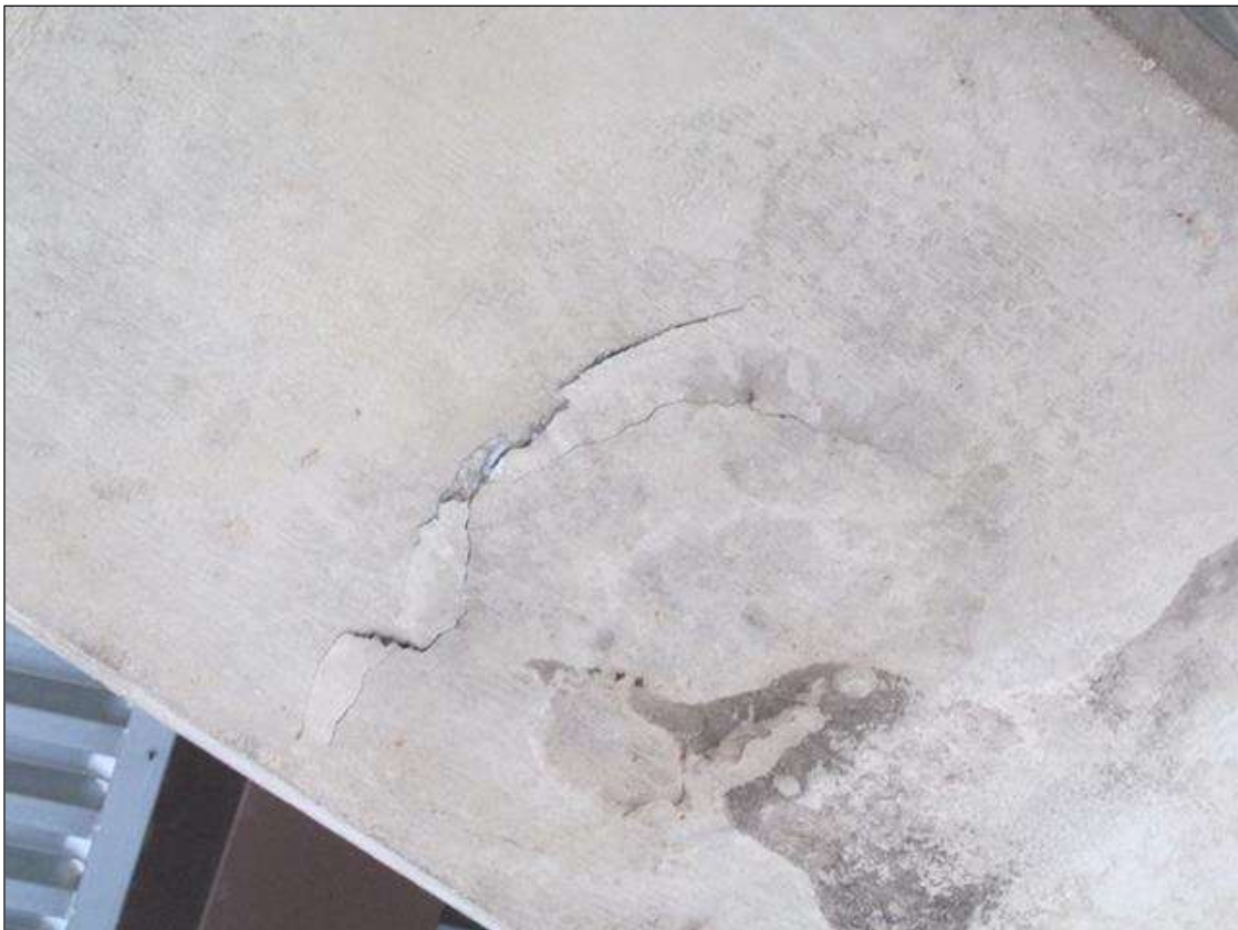
Bent 2 Cap : 6 Feet of Cracking (RC and Other): Width 0.012-0.05 in. or spacing of 1.0-3.0 ft.
