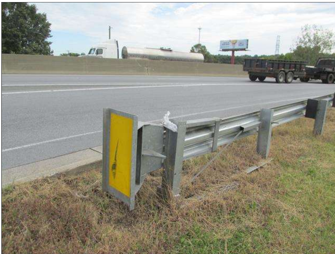
GR END AT SE CORNER. GR AT NE & NW CORNERS TIED TO EXTENDED RUNS.
