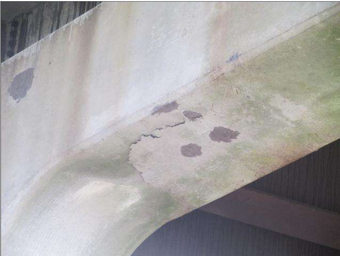
Bent 4 Cap : 6 Feet of Cracking (RC and Other): Width greater than 0.05 in. or spacing of less than 1 ft. SPALLING
